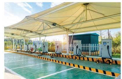
A combination of level 2 and 3 chargers provides challenging power quality issues which can be mitigated with proper transformer selections.
